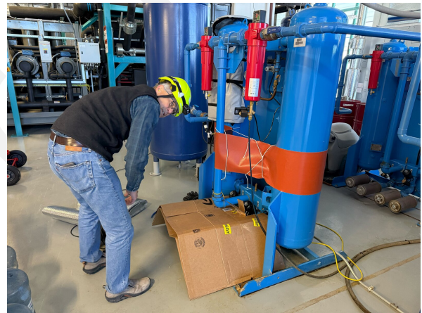
FIGURE 12: AIR-01. The compressed-air dryers at Level 1, whose freezing in August stopped the air: the towers with their exhaust and drain lines, and the insulating jacket being fitted (2025-08-23 and 2025-08-26).
