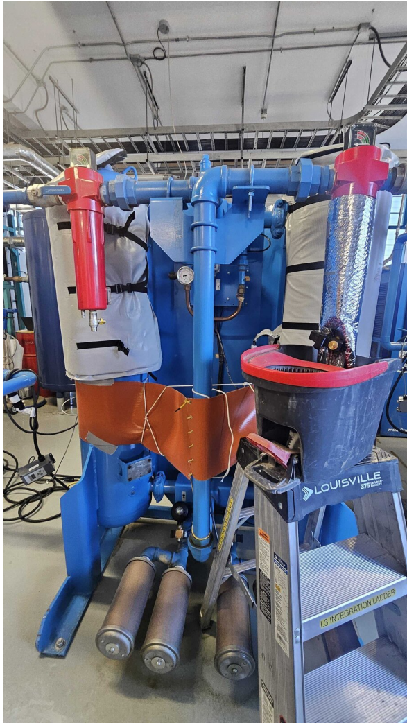
FIGURE 12: AIR-01. The compressed-air dryers at Level 1, whose freezing in August stopped the air: the towers with their exhaust and drain lines, and the insulating jacket being fitted (2025-08-23 and 2025-08-26).
