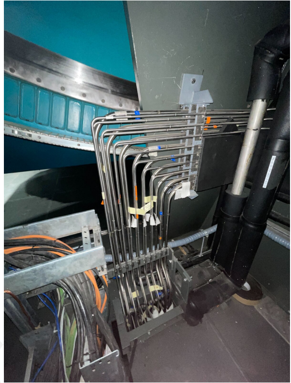
FIGURE 7: DYN-04. Refrigeration and Dynalene lines at the Top End Assembly, photographed during the June investigation of humidity and insulation in the camera region; the uninsulated runs of this kind are where the condensation found in December formed (2025-06-14).
