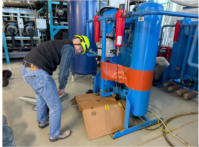
FIGURE 11: AIR-01. The compressed-air dryers at Level 1, whose freezing in August stopped the air: the towers with their exhaust and drain lines, and the insulating jacket being fitted (2025-08-23 and 2025-08-26).
