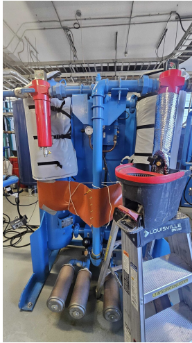
FIGURE 11: AIR-01. The compressed-air dryers at Level 1, whose freezing in August stopped the air: the towers with their exhaust and drain lines, and the insulating jacket being fitted (2025-08-23 and 2025-08-26).
